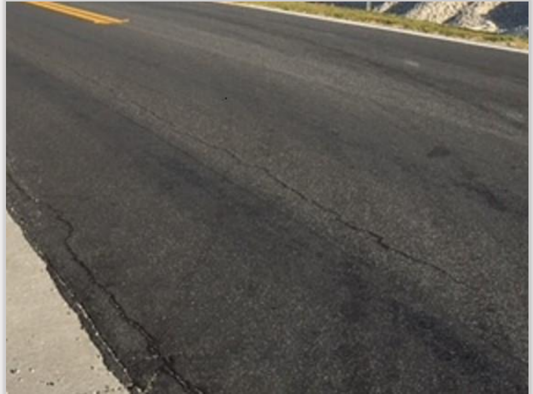
Neither Micro Surfacing nor Mill & Pave methods will stop cracks from resonating through
